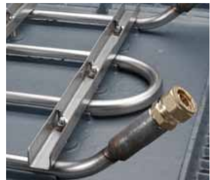
■ Cool water flows through a stainless steel tube underneath the slat.
